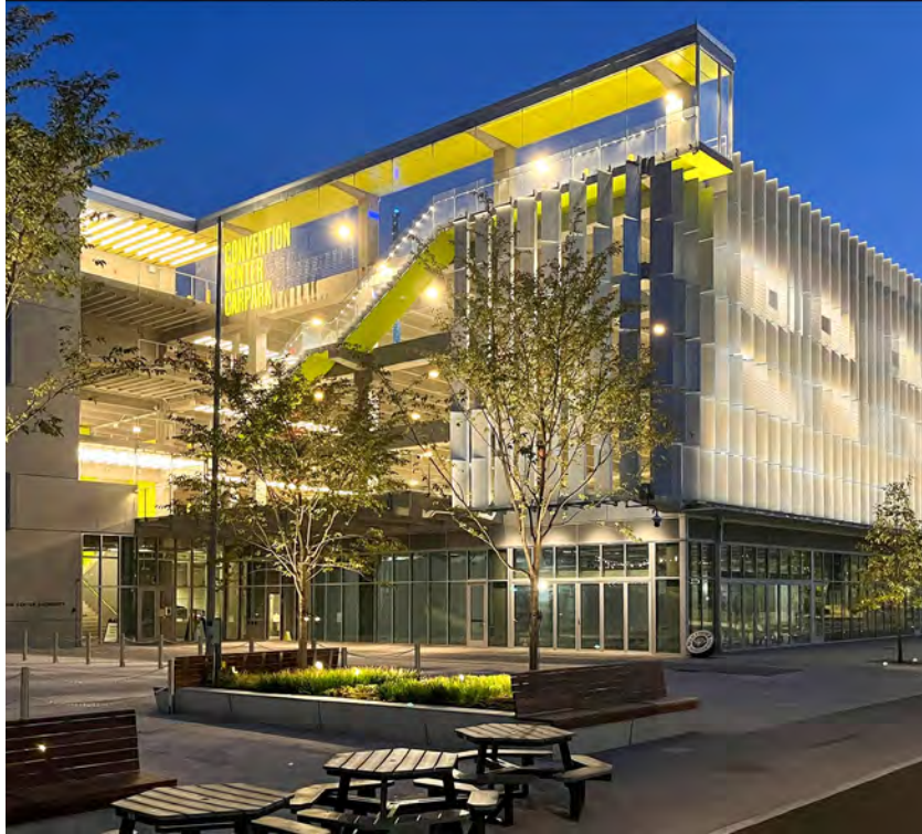
Convention Center Carpark DESMAN and Kennedy & Violich Architecture, Ltd. 2026 Apex Award, Architectural Design
